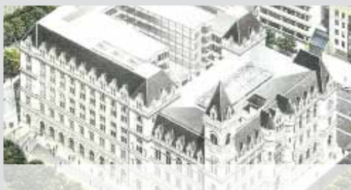
Conrad B. Duberstein U.S. Bankruptcy Courthouse, Brooklyn, New York: MBP is providing commissioning services, as well as design and construction management services for this existing building to achieve the USBGC LEED Silver certification.
