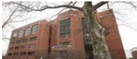
University of Virginia, Medical Research IV, Charlottesville, Virginia: MBP provided retro-commissioning services to evaluate the operation of the existing mechanical systems.
