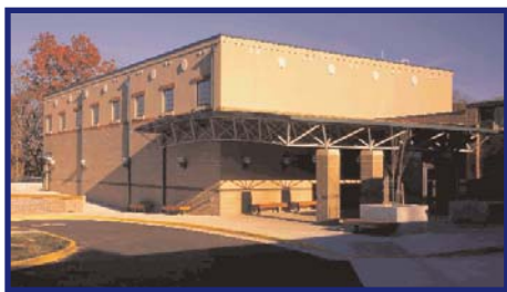
CLAREMONT ELEMENTARY SCHOOL
